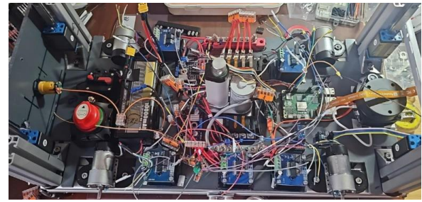
Fig. 10. Assembly and wiring components.
